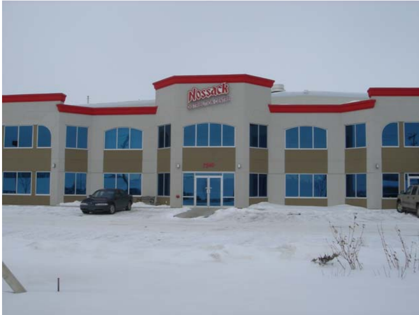
Articulation in the roof line breaks up long horizontal lines.
