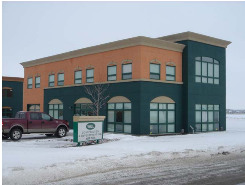
Business identification sign utilizes the same architectural vocabulary as the building.
