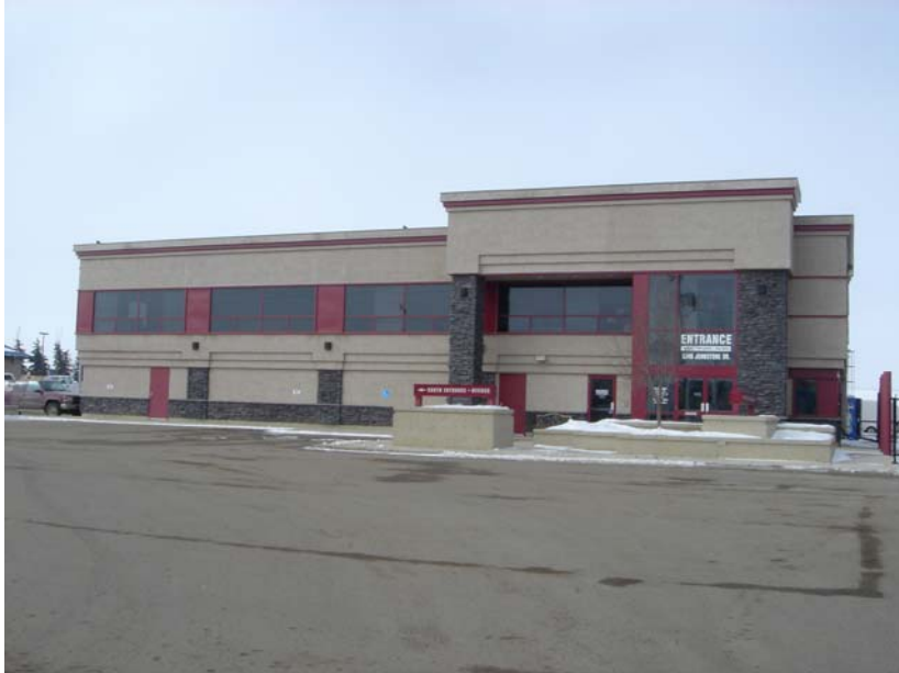
Contrasting colours and materials used for trim and accent provide visual interest.
