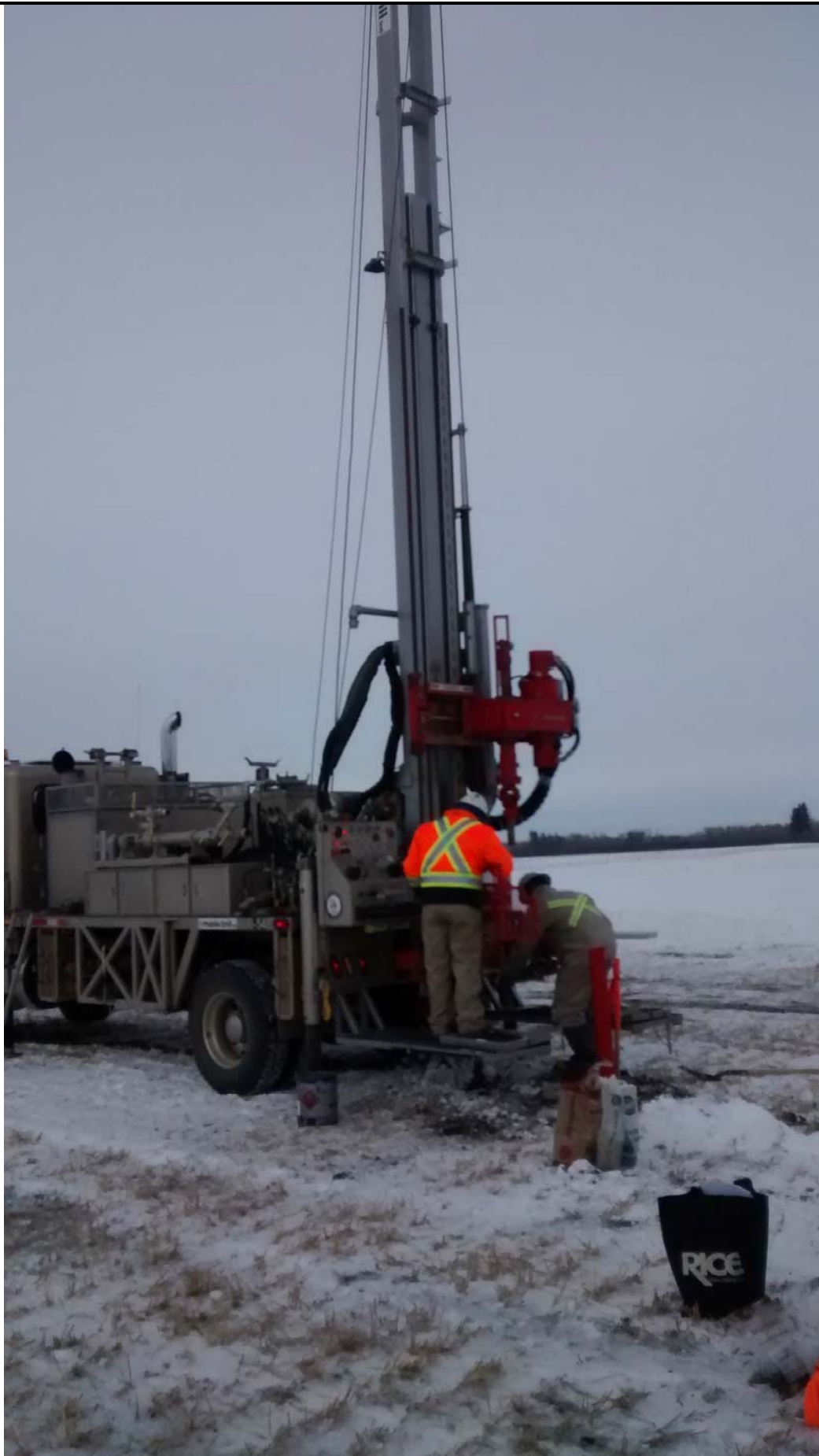
Drilling borehole at MW14-5a
