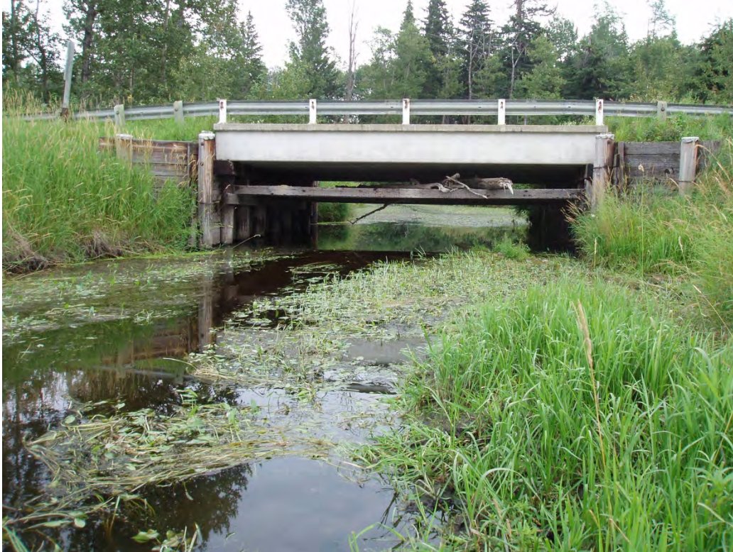
↓ Photo 13: View downstream to the Range Road 26-3 bridge, Whelp Brook (Site 4), August 7, 2013. The rafted woody debris under the bridge is indicative of high water.
