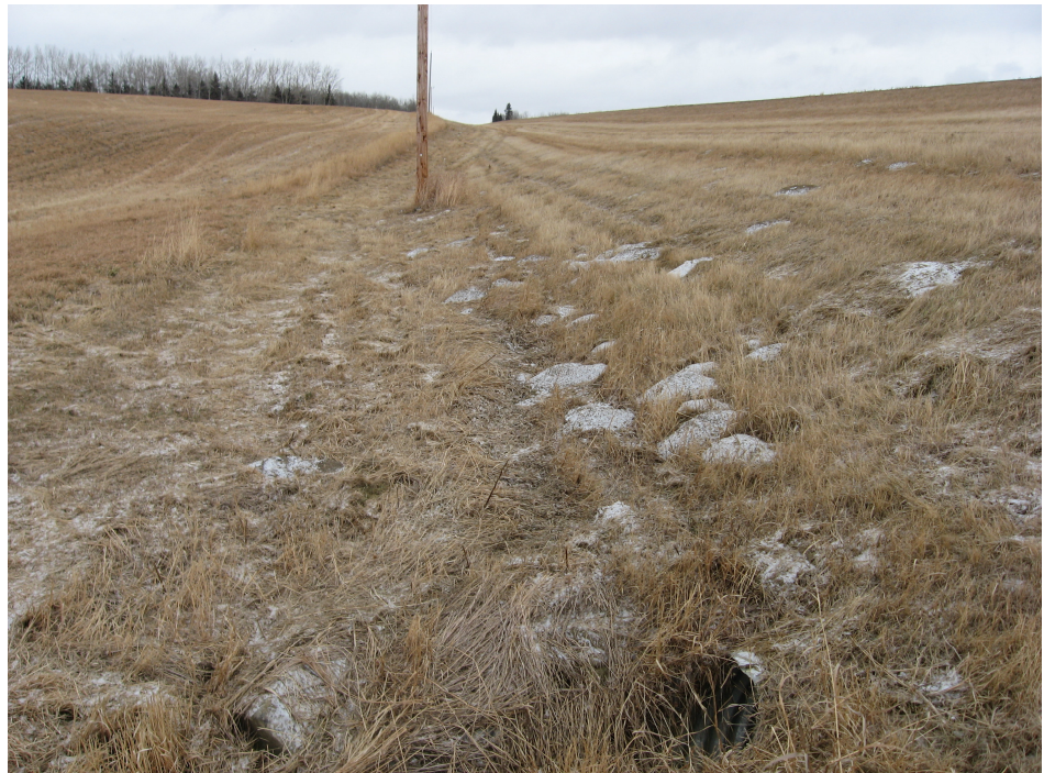
Photograph #6 Looking east on the North side of Rainy Creek Road near the culvert inlet.
