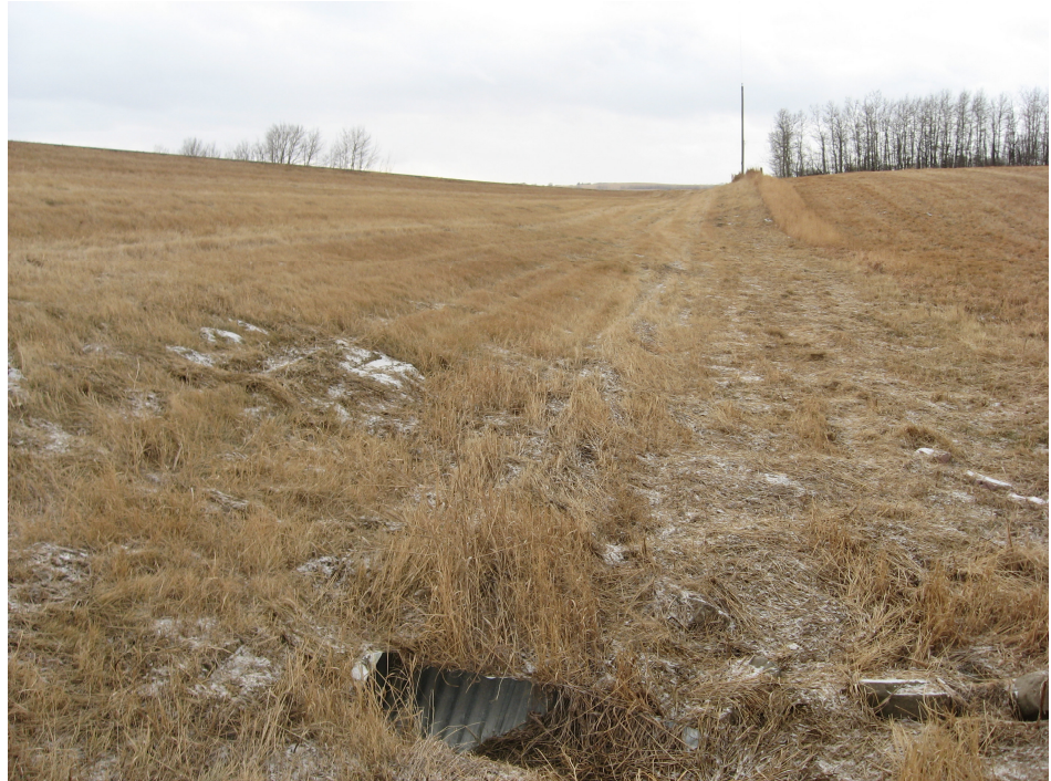
Photograph #5 Looking west on the North side of Rainy Creek Road near the culvert inlet.
