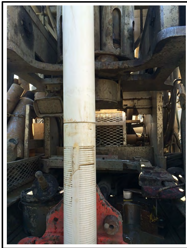
Installing the screen at SE-1 on August 4, 2016
