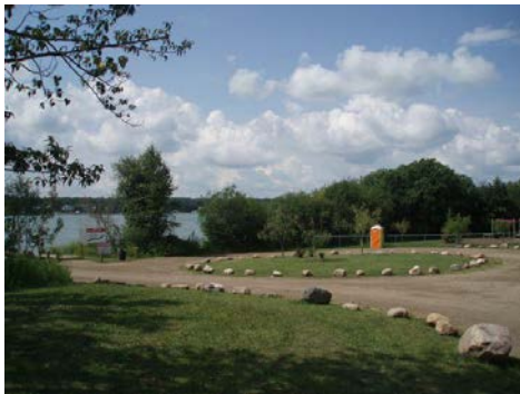
Large diameter (36 metres) turn around/stacking lane
