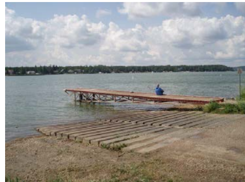
Single launch with double row of concrete pads. Metal dock 12 metres
