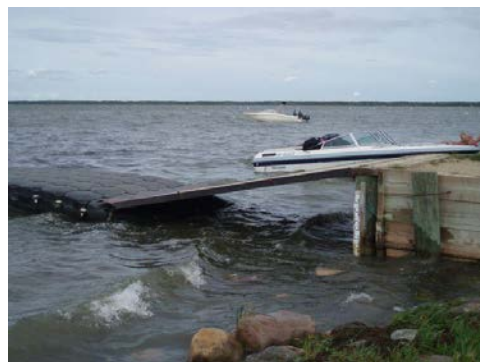
Dock attachment to allow for fluctuating water levels
