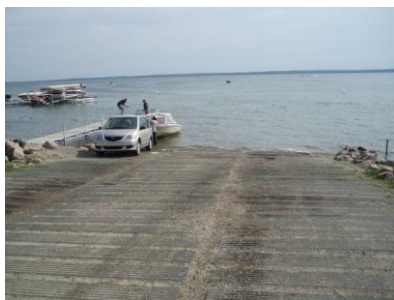
Double launch with triple concrete pads
